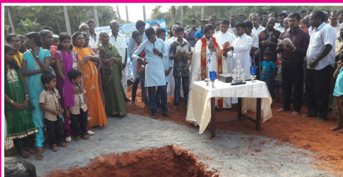
Foundation Stone for Soosaipuram Church 13.08.2017
