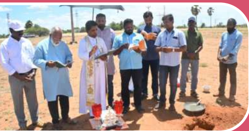
Foundation Stone Laid for the Community Hall at Kayathar, 2023 October 06
