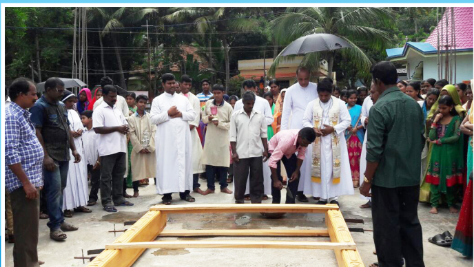
KAZHUVANTHITTAI CHURCH CONSTRUCTION RESUMED - JULY 03
